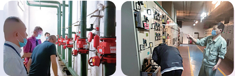
Construction Safety Thematic Training Program at Shanghai Wujiaochang Branch Store
